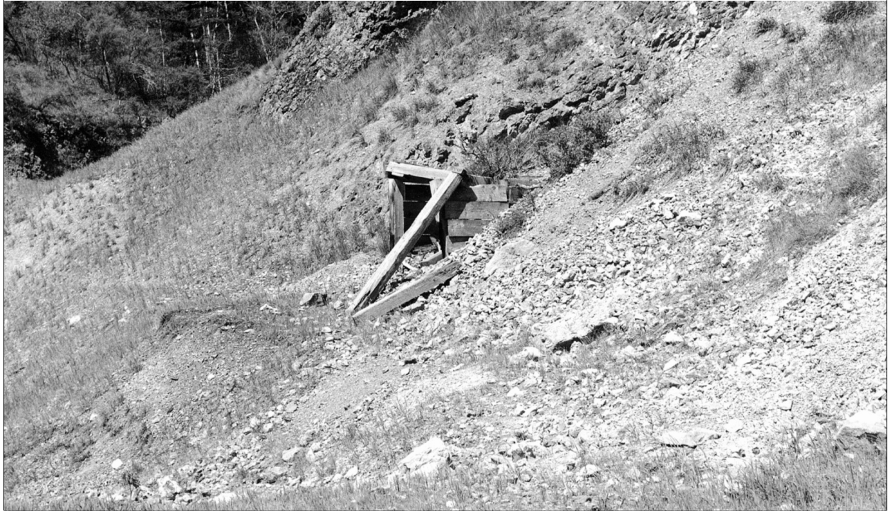
Figure 138. Caved Fall Creek Mine adit, June 2, 1997. Photo by Charles Horsburgh, BLM.
